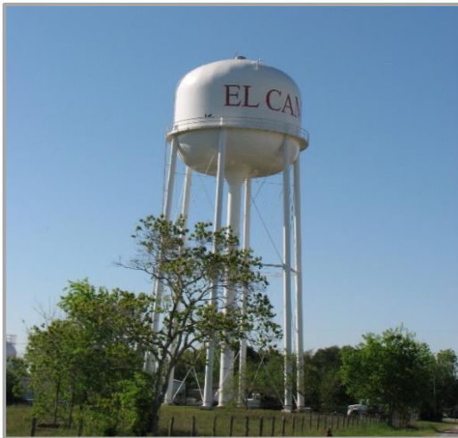
Water Plant #3 (Kentucky Plant)
